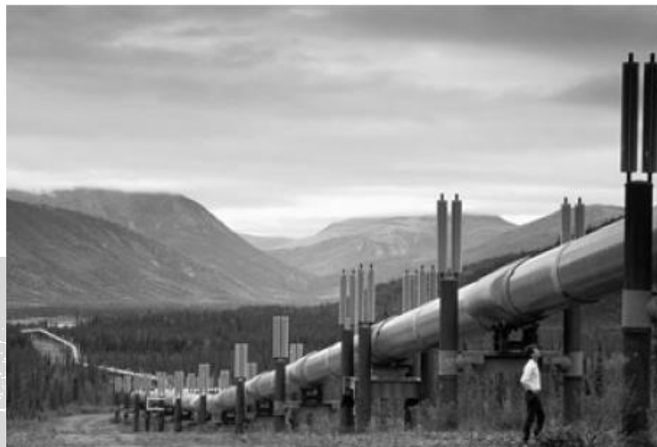
The Alaska Pipeline
